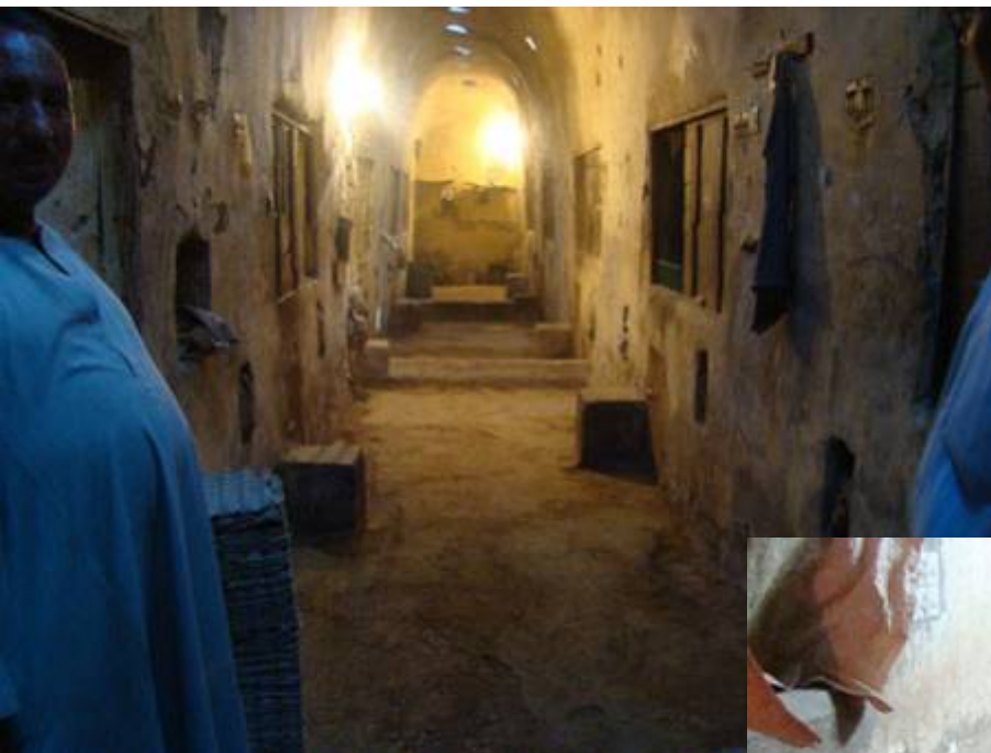
Left: Dome shaped, interior capture. Photo: M. Ali Abd-Elhakim.
