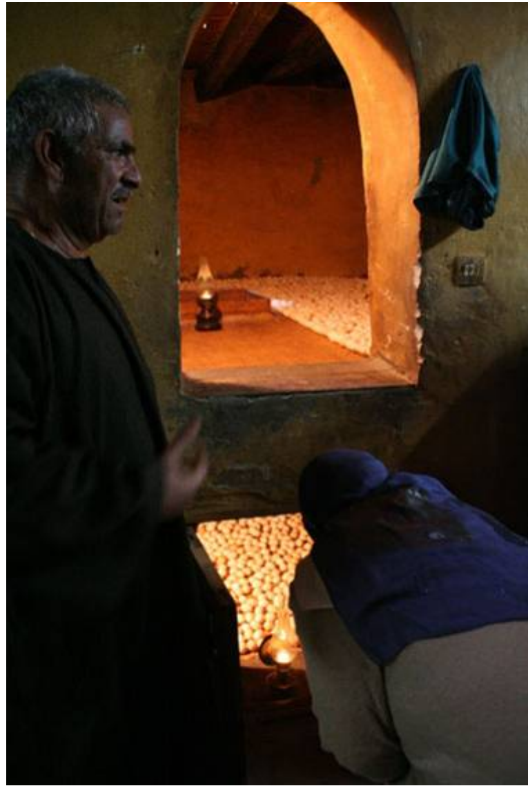
Above: Each egg house ( bait or oven) is divided into two levels (upper and lower units) and has a separate entrance. Photos: Lenny Hogerwerf.
