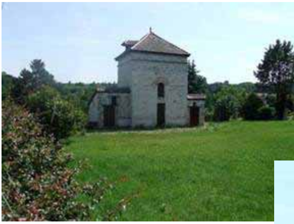
Left: At the entrance of the village of St. Sylvestre, there is a wonderfully restored pigeon tower.
